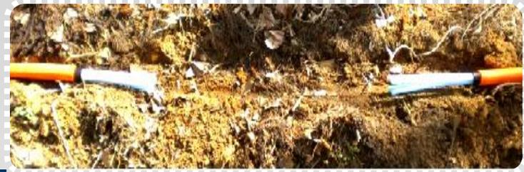
**1** Peel off outer sheath of MD after cutting off the impaired part
