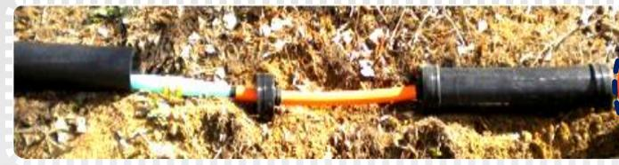
**2** Insert the MD repair socket and reconnect the cable
